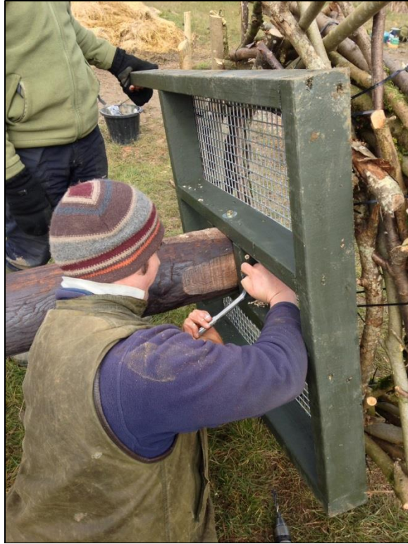
M10 coach screws are used to fix the frame. to the pole.
